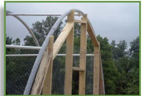
the vertical studs about 40 inches from the bottom. After the framing is complete, cover the ends with poultry wire. Drill 2½-inch holes in the base of each end frame, and drive the rebar (short for "reinforced bar") through the hole to secure the end in place. Additional bracing may be needed to help stabilize the structure during high winds and snow.
